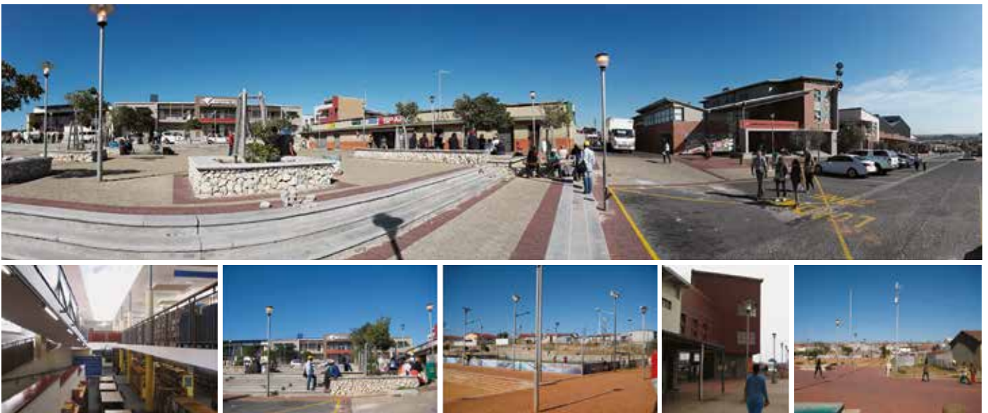
Figure 5. The panoramic photo shows Harare Square, the core of the Harare project. The small photos show – from left to right – the interior of the library, a detail of the Harare square, a soccer field space, one “Activity Box” next to the station and a portion of the Urban Park.
