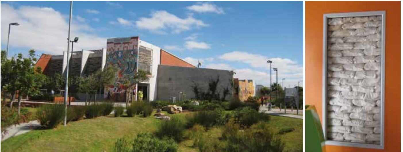
Figure 4. Photo of the Manenberg Human Settlement Contact Centre's main façade – on the left – and of the “eco-beam & sand technology” used – on the right.
