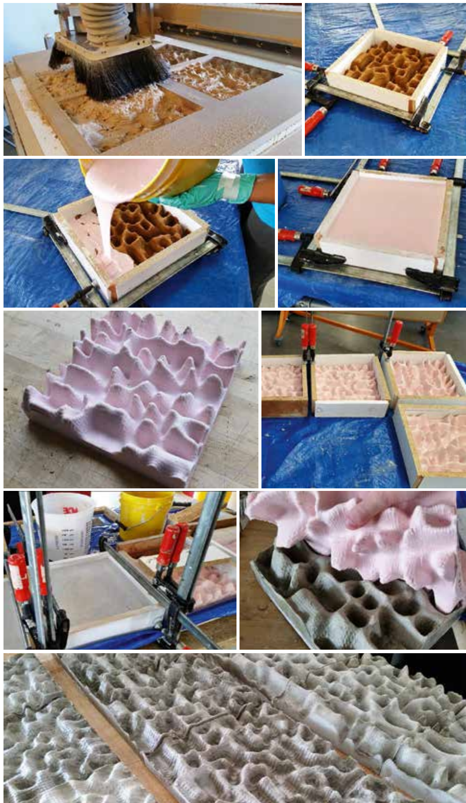
Figure 9. Fabrication workflow: Selected 25x25 cm [9.84 by 9.84 in.] surfaces were milled in MDF and sealed with shellac (1-2), silicone rubber was poured over the MDF to create the master molds (3-5), master molds lubricated and concrete poured over (6-7), removal of complex molds from surface (8), and final sixteen tiles delivered for aquarium experiments (9).
