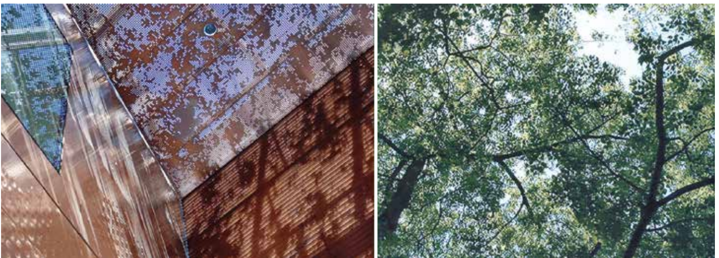
Figure 1. De Young Museum (Herzog & de Meuron) perforated copper panels and forest canopy effect.
